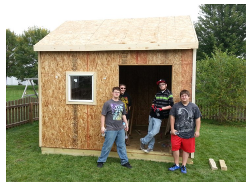
Adrian Smith, Cory Birmingham, Daniel Eaton and Tyler Clark worked to construct this shed as a part of Saydel's Building and Construction class.
