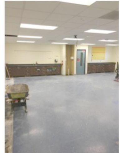
Construction work in Room 118 is at the mid-point of completion.
